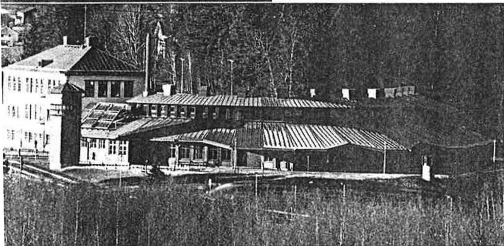
Green Building Challenge '98 is a competition and an international collaboration which has the aim of developing environmental evaluation of buildings. The results will be published this month at a conference in Vancouver. The Swedish school building Laggarbergsskolan at Timrå (Sundsvall) is one of the twelve Swedish projects selected for the competition.
