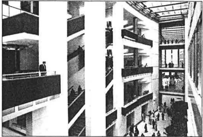
A powered smoke and heat exhaust system has been applied in the recently-opened EuroParliament building in Brussels.
