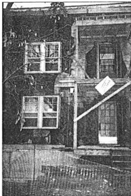
After getting efficiency renovation suggestions as a part of an energy rating, the owner of this house decided to replace the siding.
