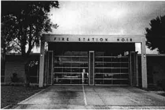
ASHRAE info: Photo #1 Fire Station #18 with vertical louvers located outside.
