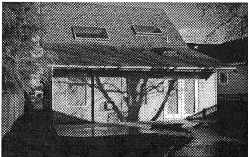
South side of house, after addition.
