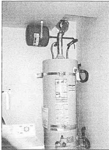
The integrated water and space heating system allows redirected hot water from the water heater tank (left) to be used to heat Village Green homes. The small incremental cost to use the water to heat the home is far less than the comparable cost of an electric heat pump. The air handler (right), with heating and cooling coils, can be located anywhere in conditioned space, preventing unnecessary duct leakage.
