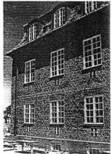
The installation of vent convectors can be made so it suits the appearance of the building. In this picture to the right four small grids with brick in between have been used instead of a standard grid. An exhaust air system with a heat pump, and 38 vent convectors in the outer walls, was in this case considerably cheaper than installing an exhaust – and entrance air system with a heat exchanger for the heat recovering.
