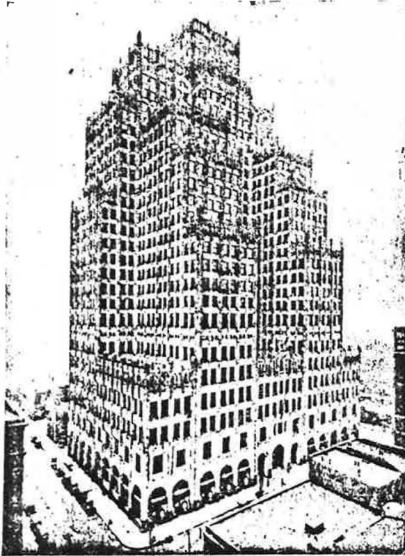
FIG. 3. SOUTHWESTERN BELL TELEPHONE BUILDING, St. Louis, Mo.
