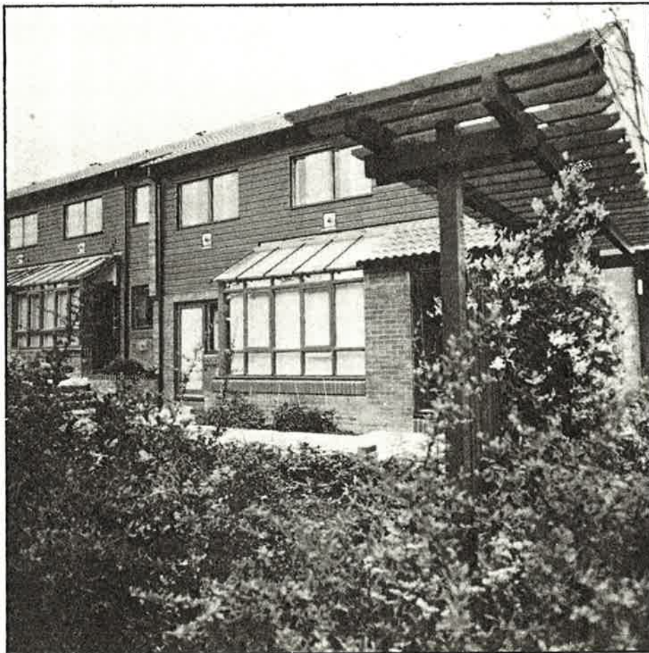
The development at Giffard Park is in four terraces.
