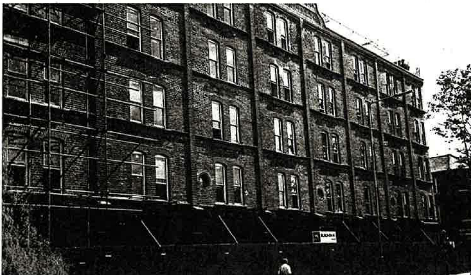
Victorian flats undergoing energy efficient refurbishment in London.
