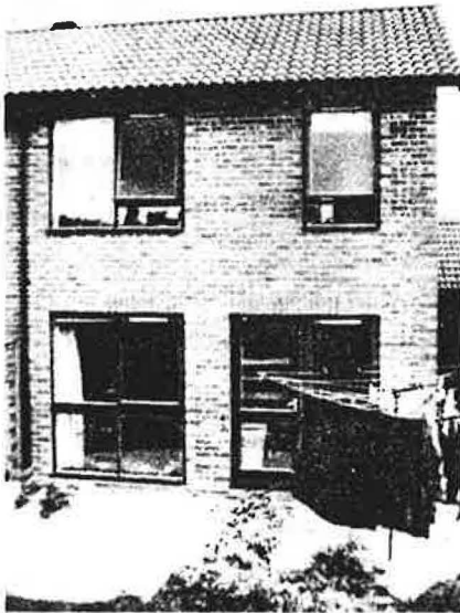
Photograph 3 Oak Farm Road - South Face
