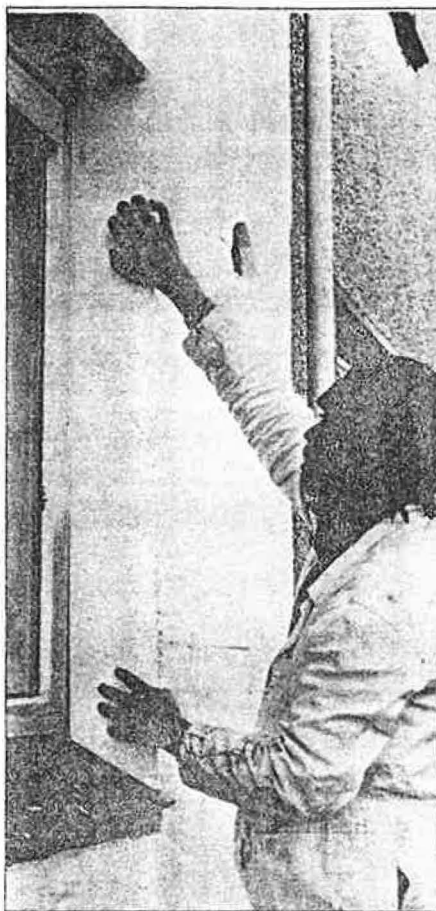
Warm coat: external wall insulation cuts heat loss to give a U-value of 0.45 \text{ W/m}^2\text{K}
