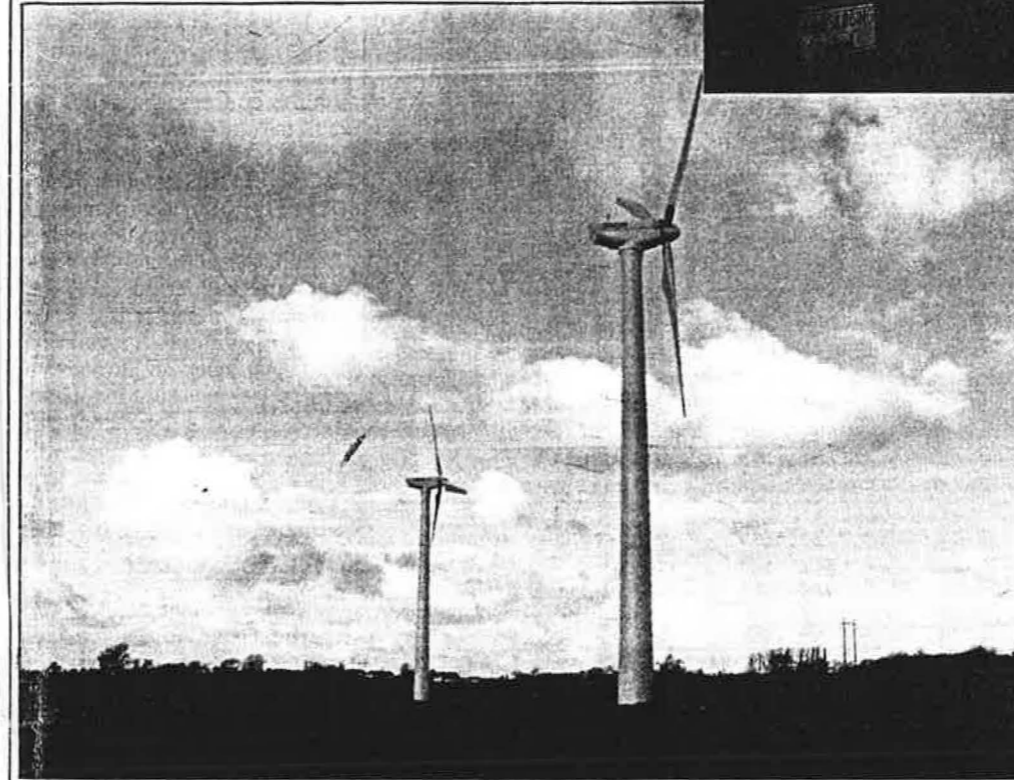
Above: The two 200 kW windmills produce 783 MWh annually.
