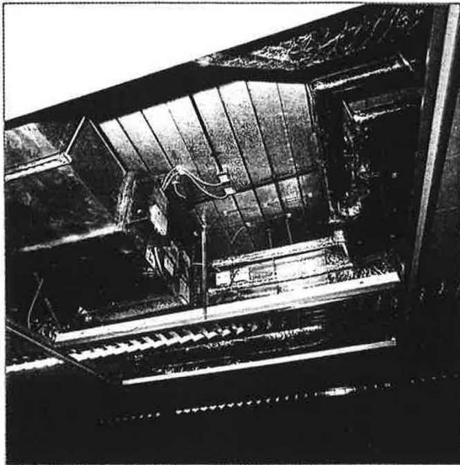
Above: Fan-powered mixing box.
