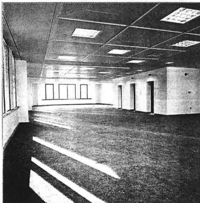
Above: High induction diffusers are used to combat dumping.
