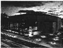
Johnson Controls was part of the design team for the 20,000 seat Bradley Center sports complex in Milwaukee, WI. Our own employees now service and operate the HVAC mechanical equipment, temperature control, lighting, fire alarm, closed circuit television systems we designed and installed.
