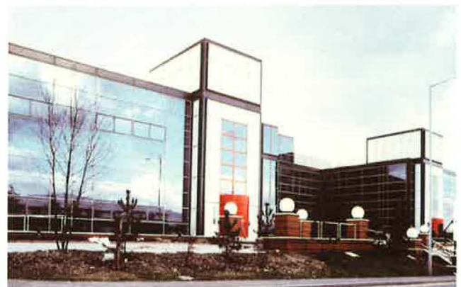
Figure 2 Example of a highly glazed, high-tech mixed-use building
