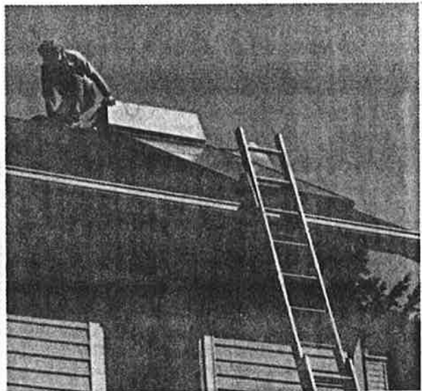
The "Copper Cricket" solar water heater works on a "percolator" principle. Hot fluids from the collector portion percolate into the heat exchanger without need of a pump.
