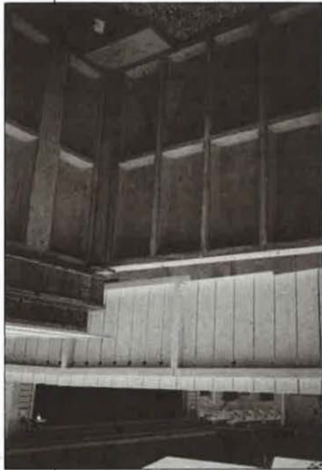
Precast concrete panels for basement walls
