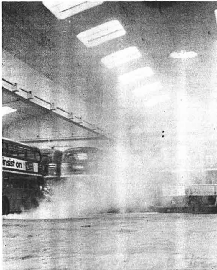
Fig. 6 Peckham garage - parking area - new ventilation scheme
