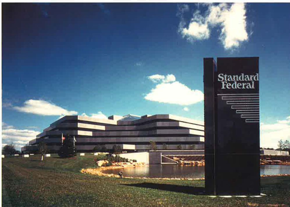
Exterior of Standard Federal Bank headquarters.
