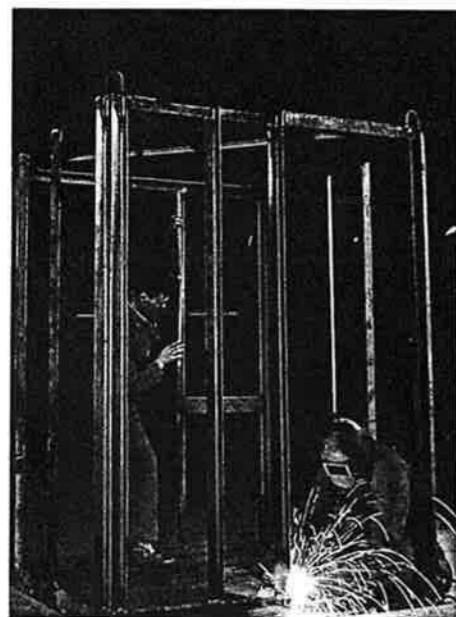
Above: light steel fabrication for the bathroom pods. Above right: the pods craned into place. Right: schematic of pod. Below right: access side of pod on a staircase. Below: a finished bathroom
