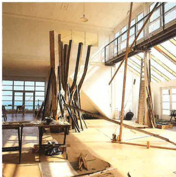
Refurbishment offers a rare opportunity to incorporate many energy efficiency measures.
