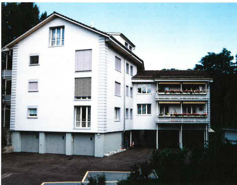
Front view after retro- fitting of the Meilen project.
