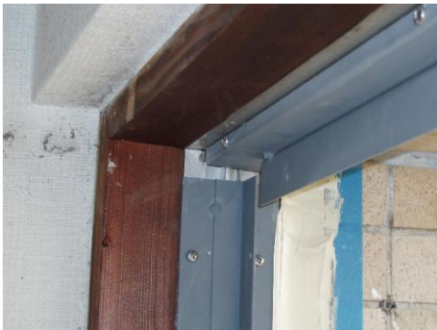
Sash retrofit of reinforced concrete housing complexes
