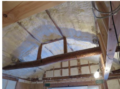
Airtight retrofit of a detached house by spraying urethane foam insulation
