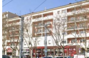
Villeurbanne (Lyon) Building 12 instrumented dwellings
