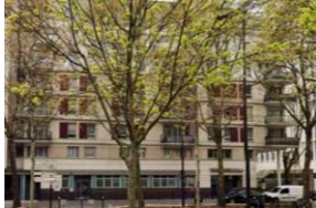
Paris Building 19 instrumented dwellings
