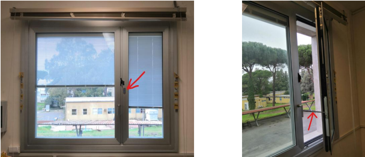
Figure 11: Front view of the new window, left, with the push-button indicated on the right sash; detail of the motorized chain to open/close the sash on the right. (Zinzi, Botticelli, Romano, & Agnoli, 2024)
